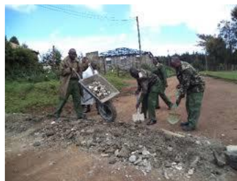
Natural road block using local fill
